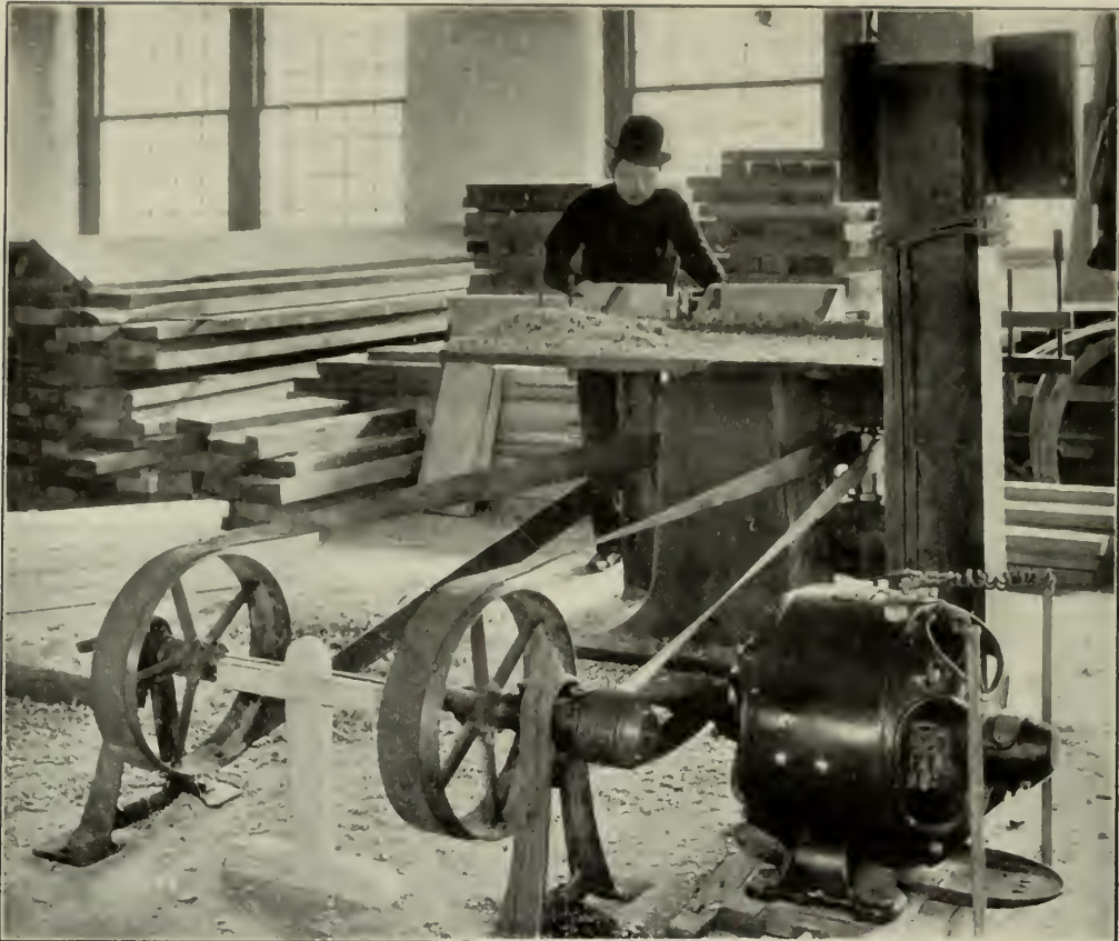
WOOD-WORKING MACHINERY DRIVEN BY ELECTRIC MOTORS.
